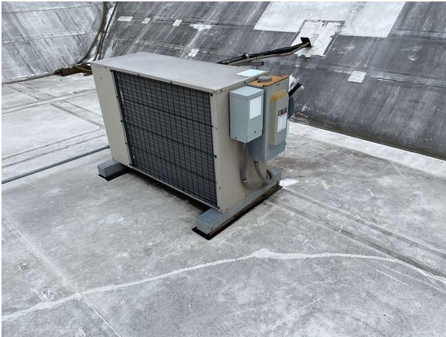
Figure D: Typical Split System Condensing Unit
