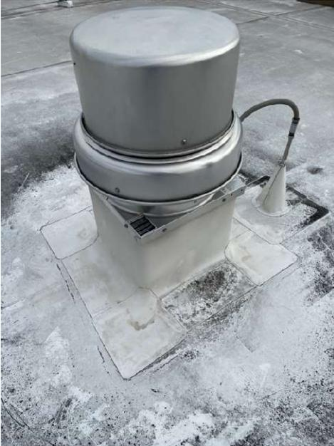
Figure A: Rooftop Exhaust Fan (Greenheck GB)
