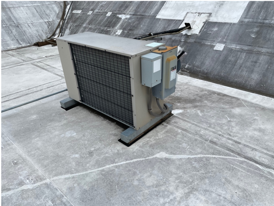
Figure D: Typical Split System Condensing Unit
