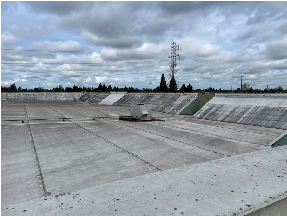
Figure B: Rooftop Surface Area
