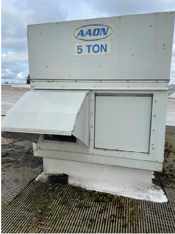
Figure C: Typical Roof Top Unit
