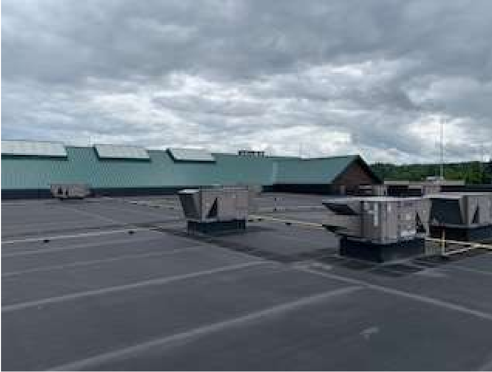
Figure A: Rooftop Surface Area
