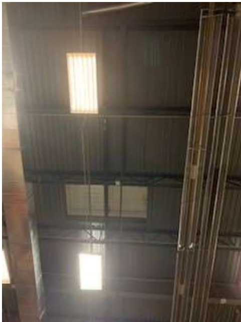
Figure F: Warehouse Lighting, 6 Lamp
