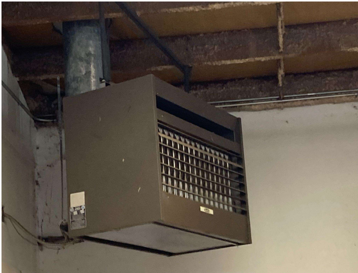
Figure U: Gas Fired Unit Heater
