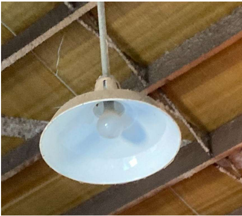
Figure E: Existing Fixture H
