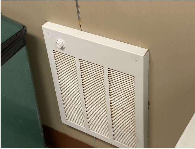
Figure M: Typical Wall Mounted Electric Heater
