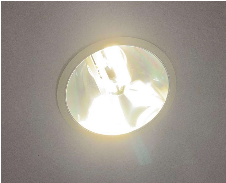
Figure D: Corridor
