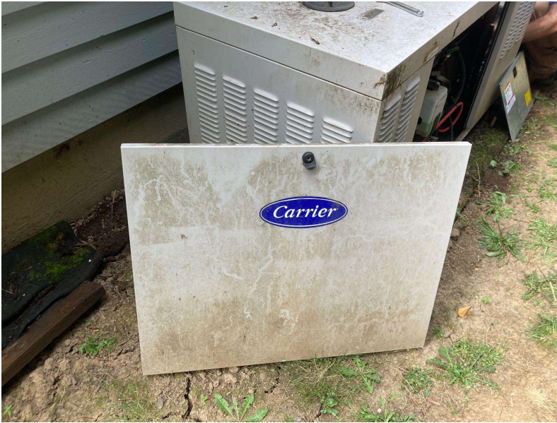
Figure F: Split System Heat Pump (Outdoor)
