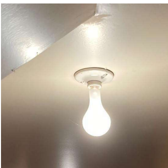
Figure C: Existing Fixture E
