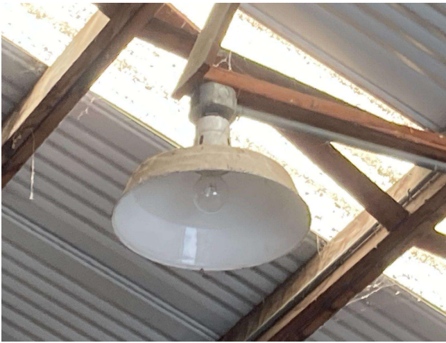
Figure D: Existing Fixture F
