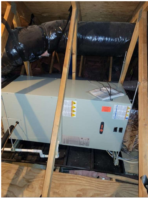
Figure C: Typical Split System Heat Pump Indoor Unit (Upper Level Attic Installation)
