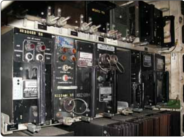
Figure 9-81. Line replaceable units in an equipment rack.
