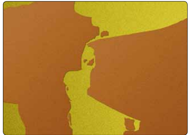
Figure 8-13. Example of poor adhesion.
