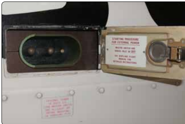
Figure 9-89. External power receptacle.
