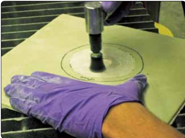
Figure 7-58. Taper sanding of repair area.
