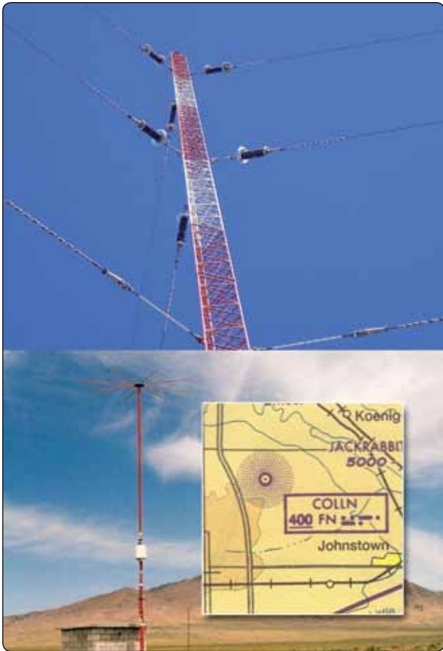
Figure 11-106. Nondirectional broadcast antenna in the LF and medium frequency range are used for ADF navigation.
