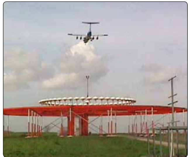
Figure 11-119. A VOR with DME ground station.
