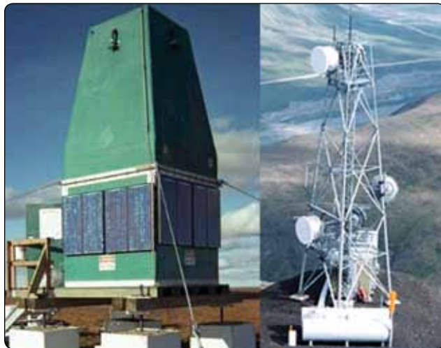
Figure 11-135. Low power requirements allow remote ADS-B stations with only solar or propane support. This is not possible with ground radar due to high power demands which inhibit remote area radar coverage for air traffic purposes.
